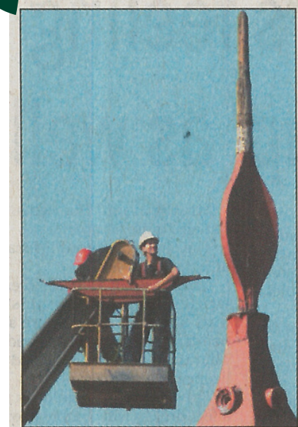
Stratford Metal Products metal fabricator Tom Newton works on the component pieces that will form the decorative accent of the Perth County Courthouse finial. Fashioned from lead-coated copper, the new piece is a nearly exact copy of the previous finial, which had deteriorated over decades. The inset above shows its removal in September. SCOTT WISHART The Beacon Herald
