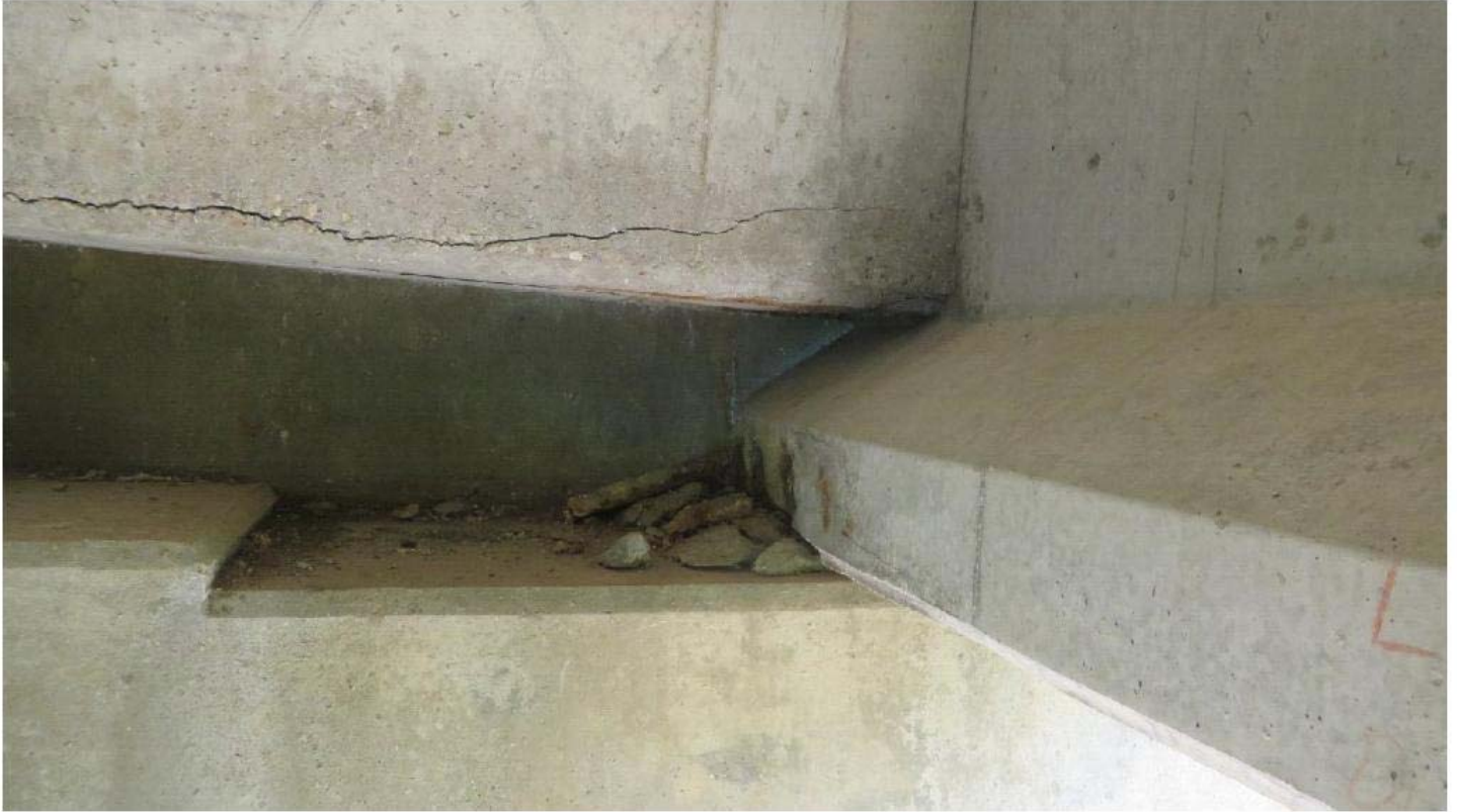
North diaphragm/girder end
